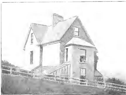
A HOME IN THE MAKING (FIRST STAGE).
